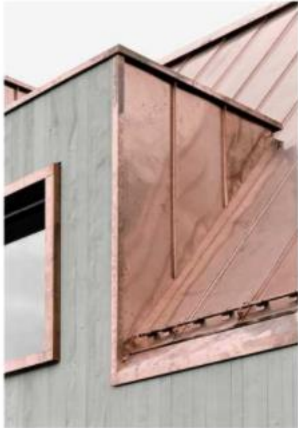
Church in Wierzbica by Mies van der Rohe Architects - Rasmus Nohrsted
